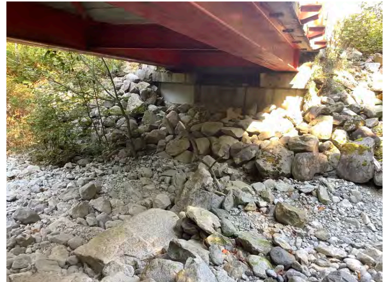
Right Bank Abutment when facing downstream
