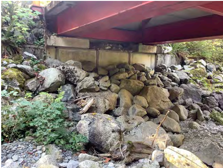
Left Bank Abutment when facing downstream
